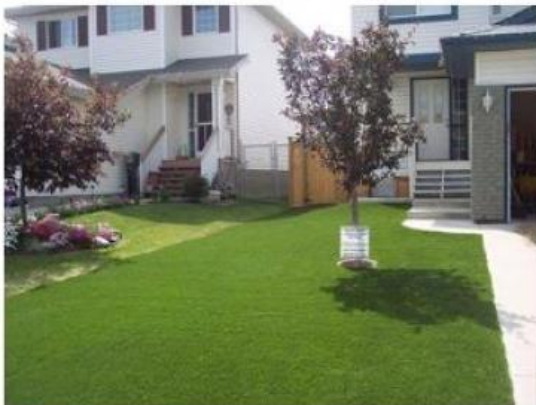
Incorrect – There should be a distinct boarder installed between the artificial turf and the neighboring natural sod.
